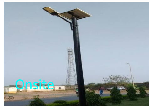
PV Solar Street Light Inside Plant
